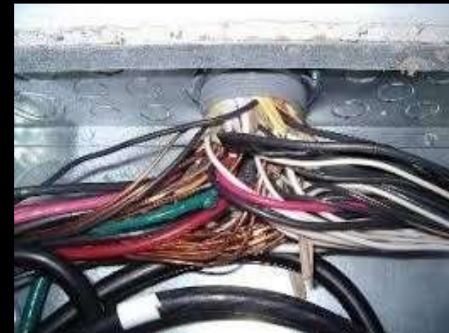
Improper wiring
