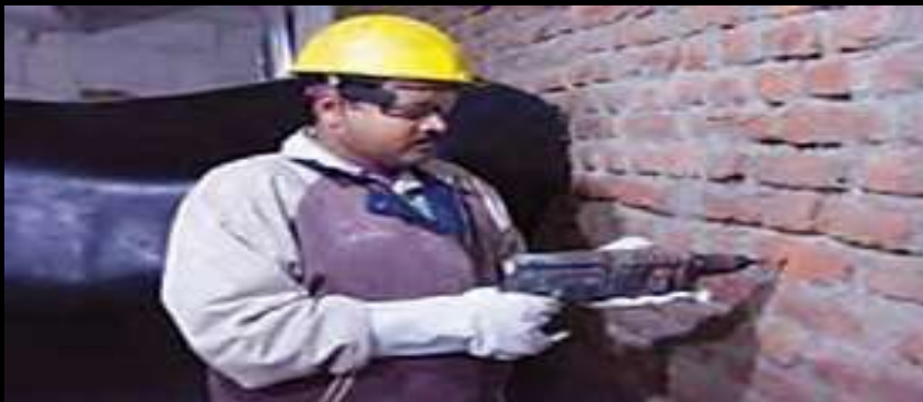
Using power drill machine
