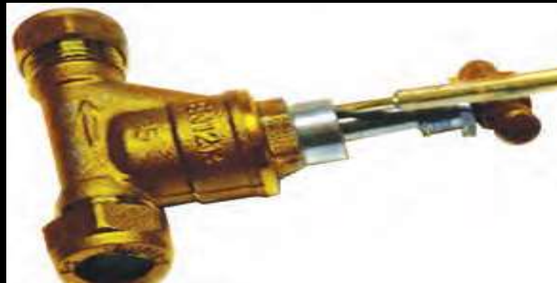
Removing bits from a gland nut
