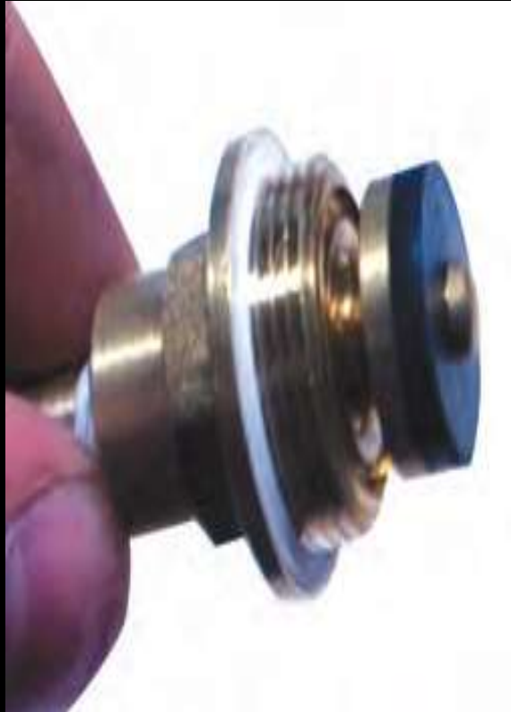
(e) Replacing the rubber washer
