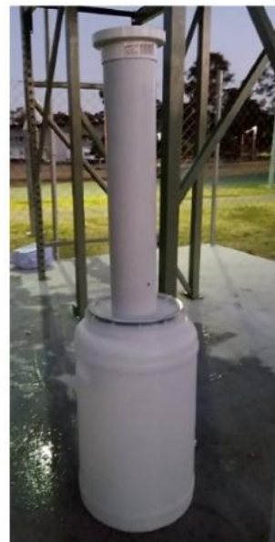
Fig. 2.15: Proper Gradation Rain Water Harvesting filter column
