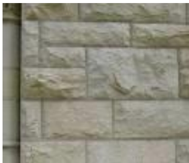
Fig.1.17: Ashlar Masonry
