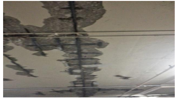
Fig 5. 8 Spalling
