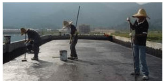
Fig.5.1: Bituminous Coating
