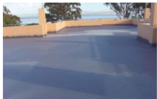
Fig 5. 3 Paint waterproofing on roof
