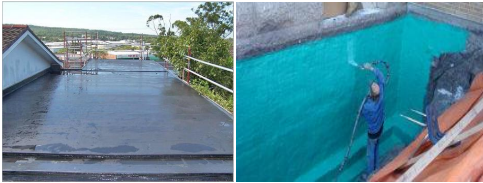
Fig.5.14 Poly Acrylic chemical coating waterproofing
