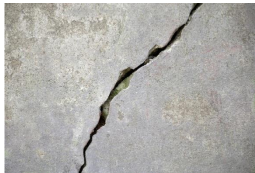
Fig 5. 4 Freeze thaw effect
