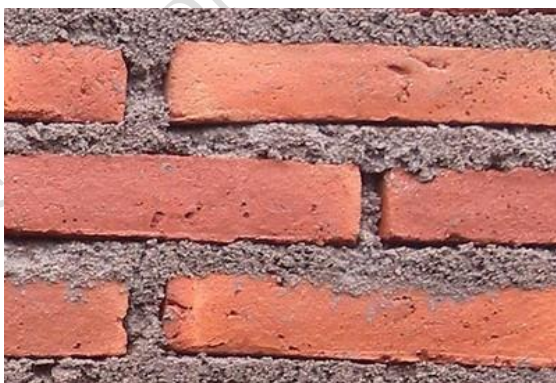
Fig.2.2: Mortar in brick joining
