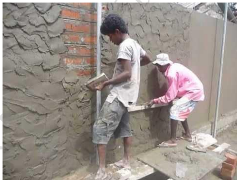
Fig.3.2 Plastering with manual labour
