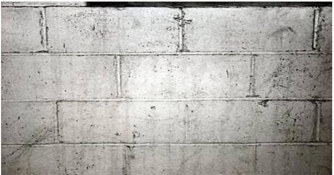
Fig.5.14: Concrete Block Wall
