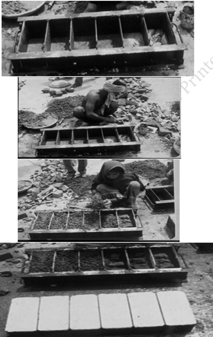
Fig.4.9: Different steps in moulding of Concrete block
