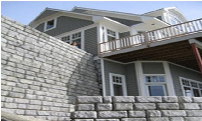
Fig.5.15: Concrete block wall in house construction
