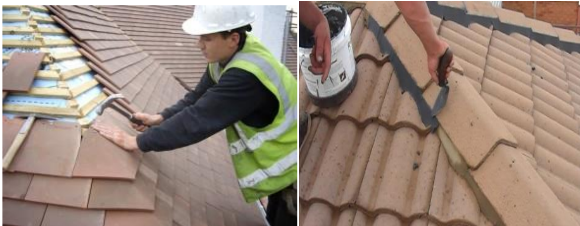
Fig 5.15 Poly Acrylic chemical coating waterproofing
