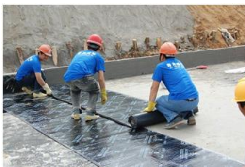
Fig. 5.2 Bituminous Membrane Laying
