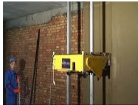
Fig.3.3 Plastering with machine
