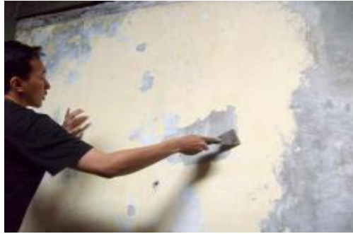
Fig 5. 3 Penetrating waterproofing
