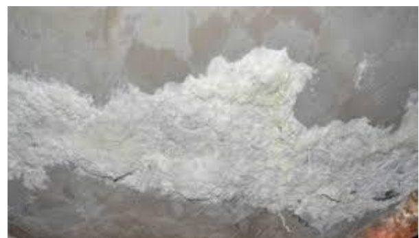
Fig 5. 11 Efflorescence
