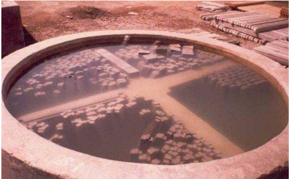
Fig.4.13: Curing Tank For Concrete Block
