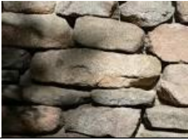
Fig.1.10: Dry Rubble Masonry
