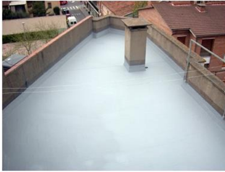
Fig 5. 3 Polyurethane Liquid Membrane
