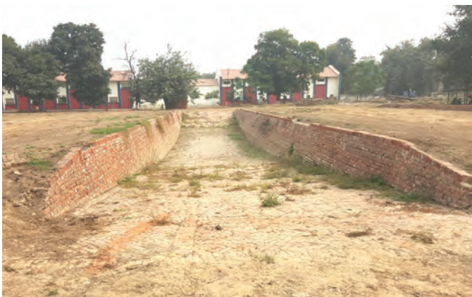
Fig. 1.9(a): Structure of bunker-type silo
