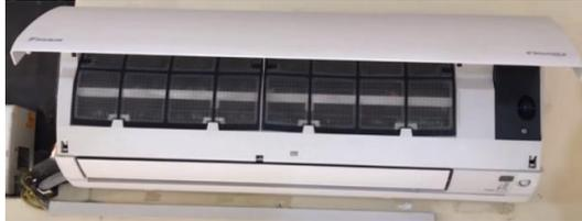
**Fig. 2.4 Open the front panel of the air conditioner**
