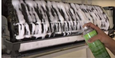
**Fig. 2.17 Applying foam onto the evaporator fins**
