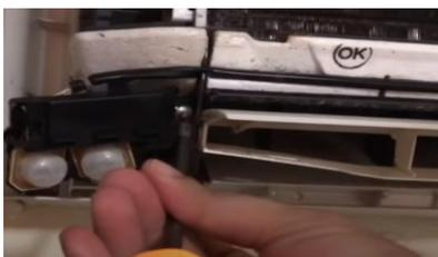
**Fig. 2.29 Unscrew the aircon tray of the indoor unit**
