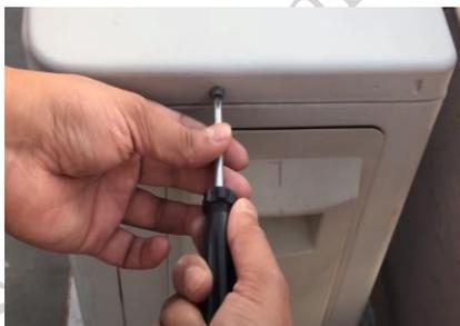
**Fig. 2.40 Removing the screw of the top panel**
