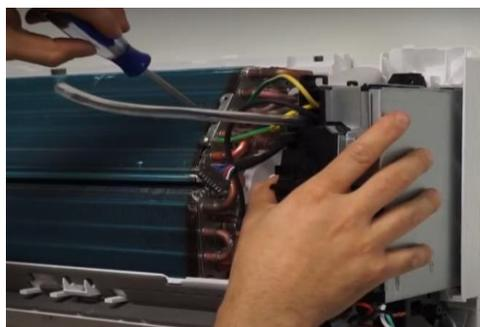
**Fig. 3.16 Removal of screw holders**
