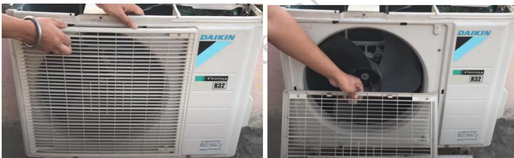
**Fig.2.43 Unlock the hooks of the discharge grille and remove the discharge grille**
