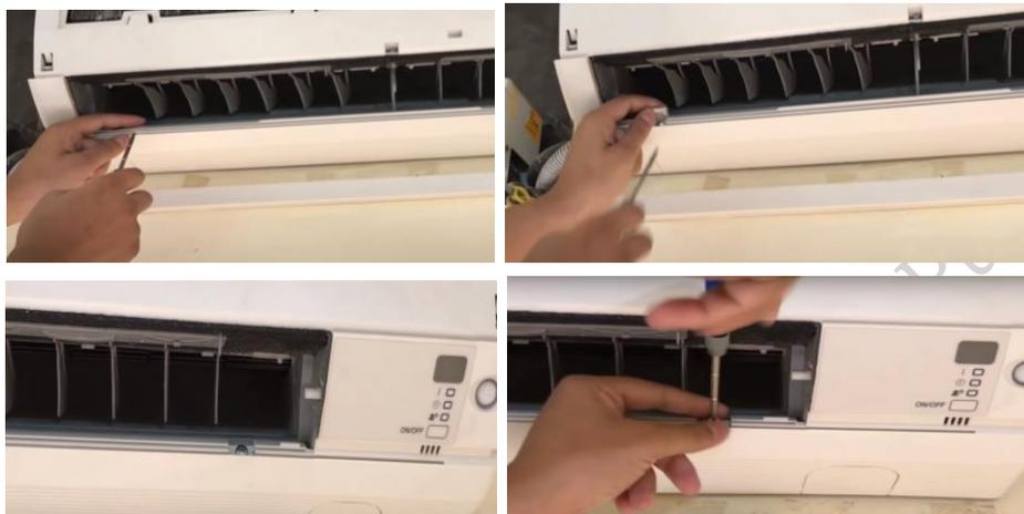
**Fig. 2.26 Removing the screws**
