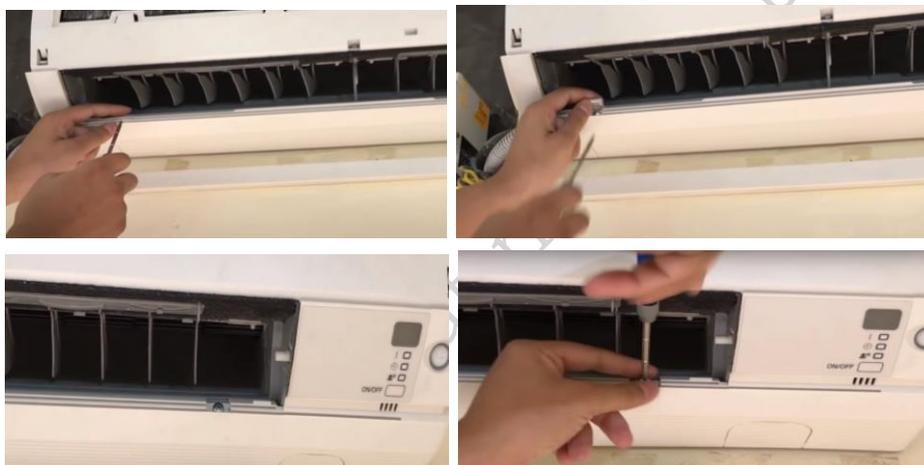
**Fig. 2.14 Remove the two screws**
