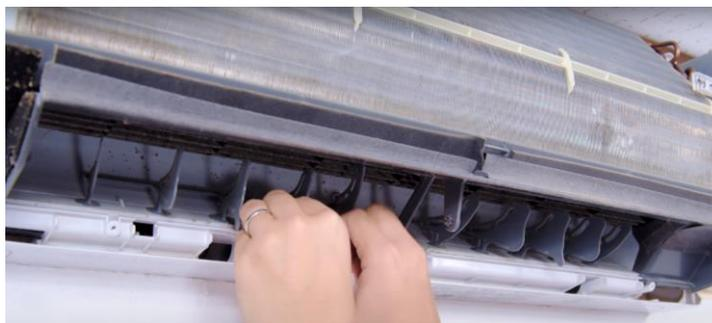
**Fig. 2.39 Removing the louvre of the indoor unit**
