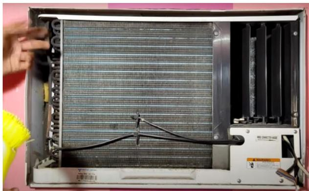
**Fig. 2.54 Remove the temperature sensor**
