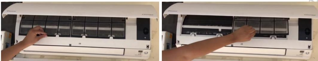
**Fig. 2.8 Unlocking the filter**
