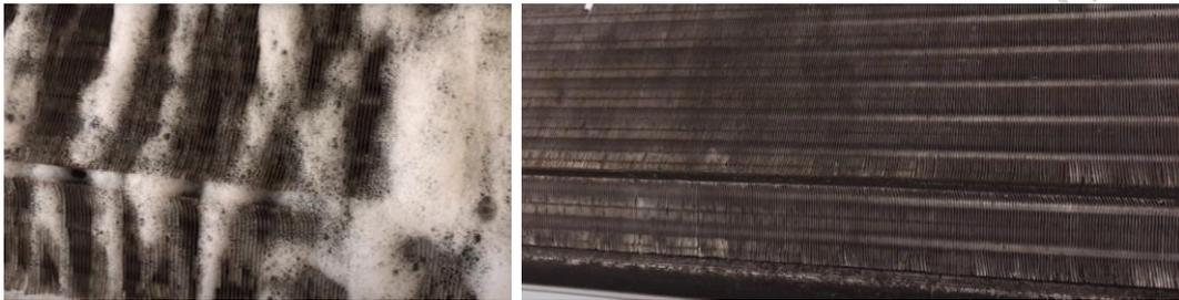
**Fig. 2.18 Cleaned fins of the condenser**
