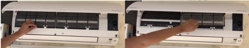
**Fig. 2.5 (a) Unlocking the first filter (b) Unlocking the second filter**
