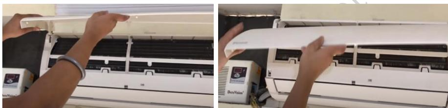
**Fig. 2.35 Sliding the left rotary shaft**
