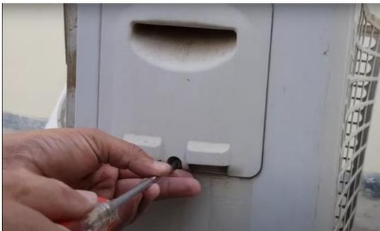
**Fig. 3.6 Detaching the connection plate**
