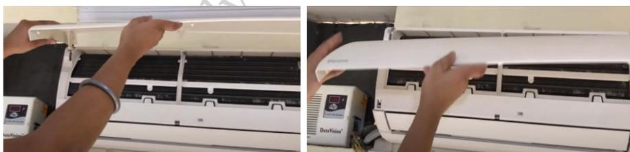
**Fig. 2.10 Sliding the left rotary shaft**
