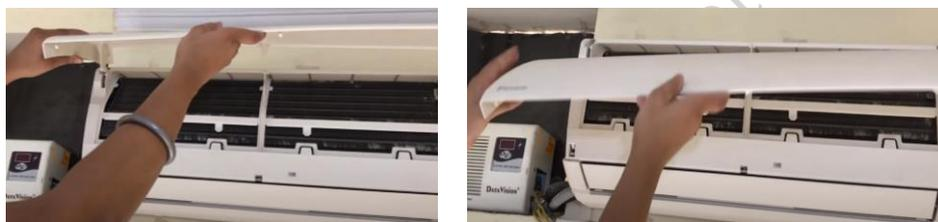
**Fig. 2.22 Sliding the left rotary shaft**
