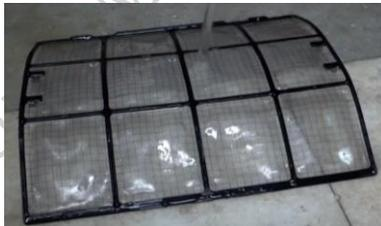
**Fig. 2.6 Removing and cleaning the filter of split AC**
