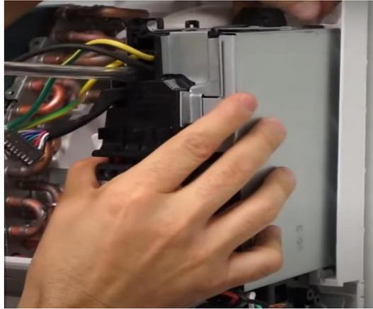
**Fig. 3.17 Removal of control box**
