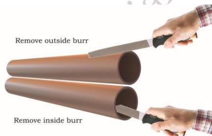
**Fig. 3.36 Reaming of copper tube**
