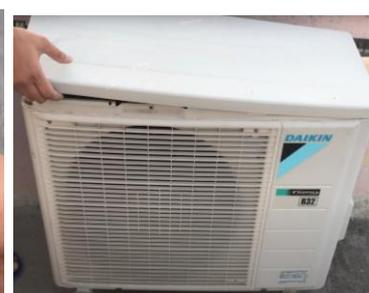
**Fig. 2.41 Lifting the top panel**
