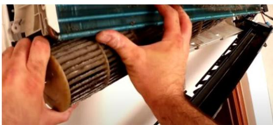
**Fig. 2.31 Removing the blower from the indoor unit**
