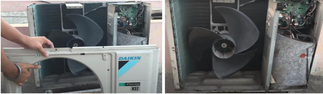
**Fig. 2.45 Unfasten the hooks, pull and remove the front panel**
