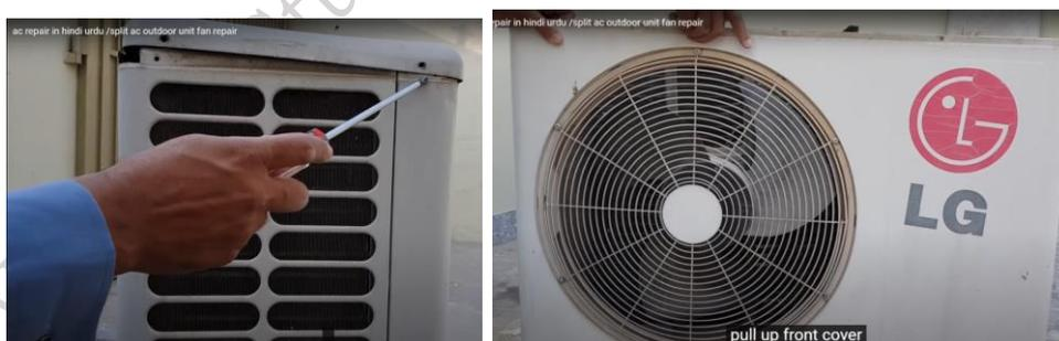
**Fig. 3.4 Removing the covers**
