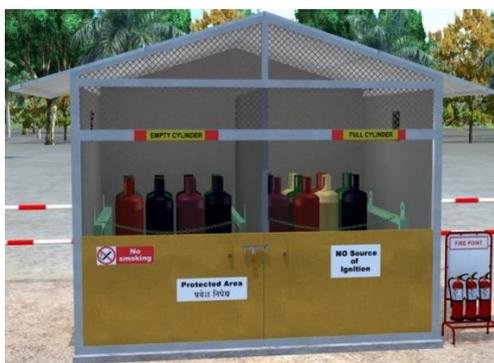
**Fig. 1.4 Storing of refrigerant cylinders**
