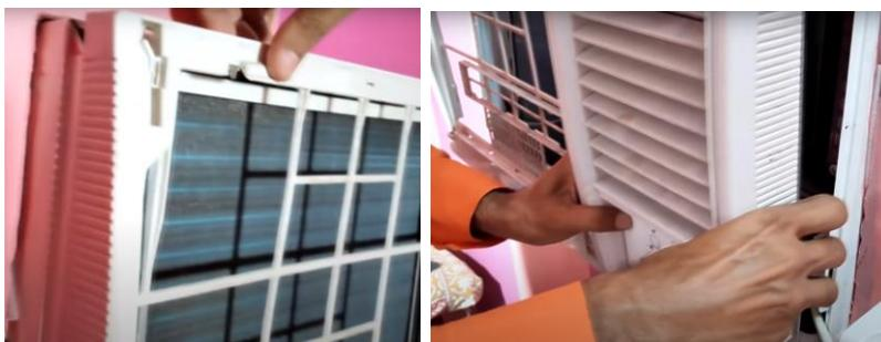
**Fig. 2.51 Detach the front panel**
