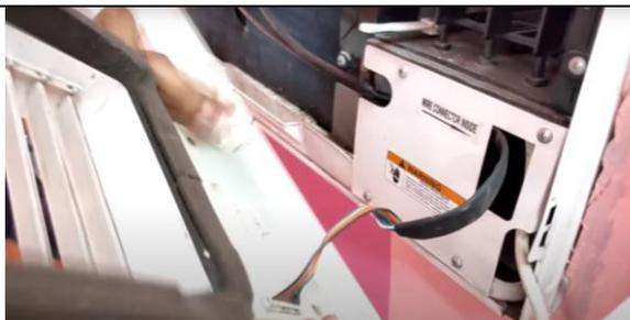
**Fig. 2.52 Remove the PCB wires**
