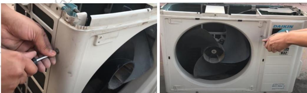
**Fig. 2.44 Removing the screw of the front panel**
