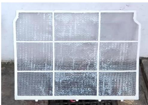
**Fig. 2.58 Wash the filter with water**
