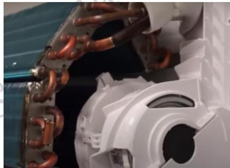
**Fig. 3.19 Removal of the cover of fan blower motor**
