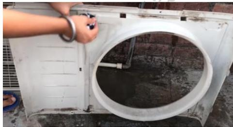
**Fig.2.47 Washing the front panel**
