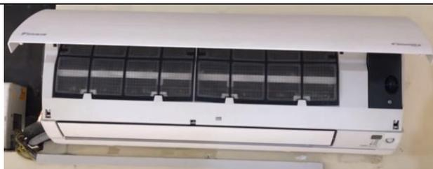
**Fig. 2.7 Open the front panel of the air conditioner**
