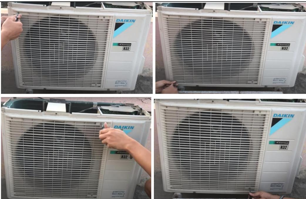
**Fig. 2.42 Remove the screws and discharge grille**
