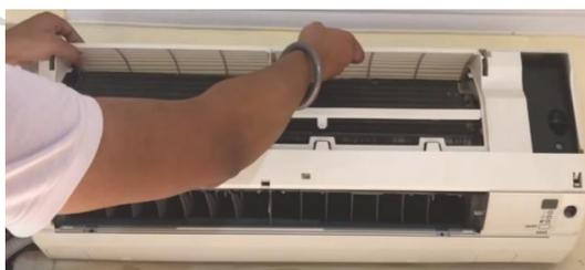
**Fig. 2.15 Unfasten the three hooks at the top**
