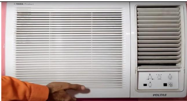
**Fig. 2.48 Removing the front grille of the window AC**
