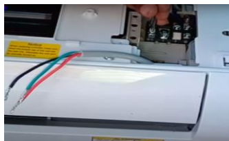
Fig.2.33 Insertion of the power cable
