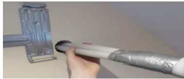
Fig. 2.54 Placing the bundle through the hole
