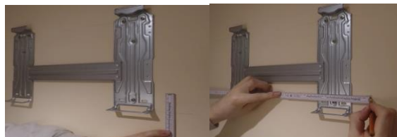
Fig.2.20 Measurement of the hole using a measurement tape
