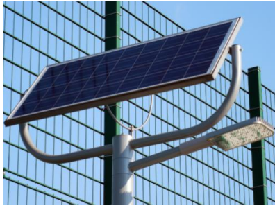
Fig. 2.17 Solar panel in street light
