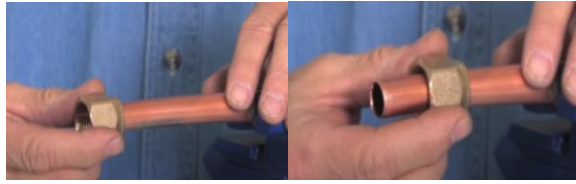
Fig.2.43 Placement of flare nut
