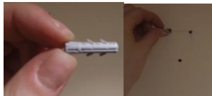
Fig.2.16 Placing the drilling anchor in the drilled holes
