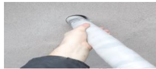
Fig. 2.55 Pulling the bundle from outside
