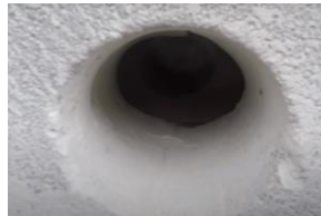
Fig.2.28 Making a final hole in the wall
