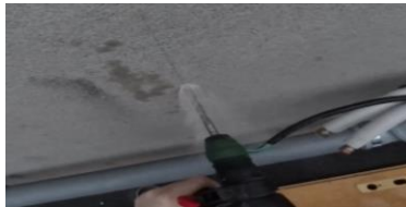
Fig. 2.59 Drilling on marked points
