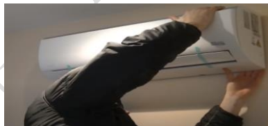
Fig. 2.56 Hanging the indoor unit onto the wall
