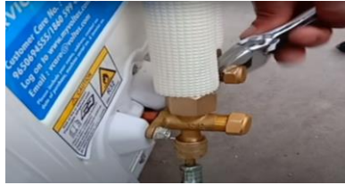
Fig. 2.67 Remove the nut of the discharge pipe
