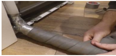
Fig. 2.53 Wrapping the insulation material
