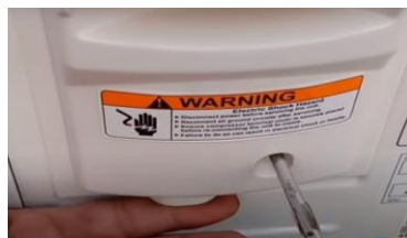
Fig. 2.70 Opening of the power box
