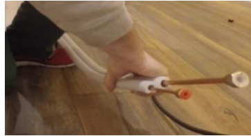
Fig.2.39 Straightening of copper pipes
