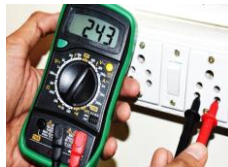
Fig. 1.76 Measuring AC voltage using multimeter
