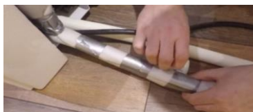
Fig. 2.52 Securing the insulation using duct tape
