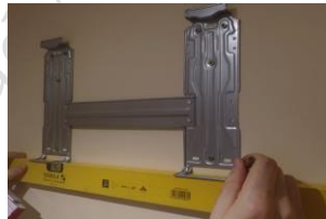
Fig.2.19 Measurement of the level using a spirit level
