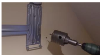
Fig.2.25 Alignment of drill bit with the desired drilling location
