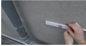
Fig. 2.58 Mark the points to be drilled
