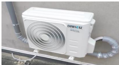
Fig. 2.62 Outdoor unit on the bracket rails
