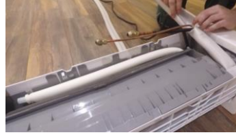
Fig.2.38 Suction and discharge pipe of the indoor unit
