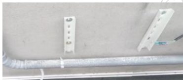
Fig. 2.60 Fixing of the bracket rails
