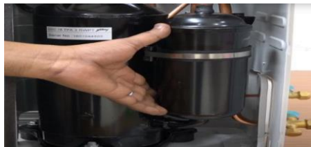
Fig. 1.39 Accumulator
