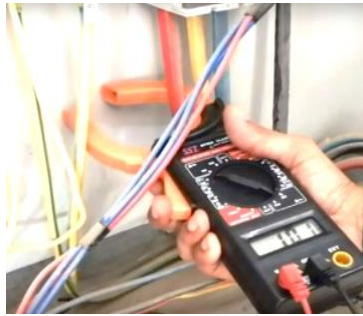
Fig. 1.68 Clamp the device around conductor
