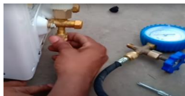
Fig. 2.65 Open the nut of the suction pipe
