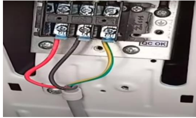
Fig. 2.71 Connection of electrical wire
