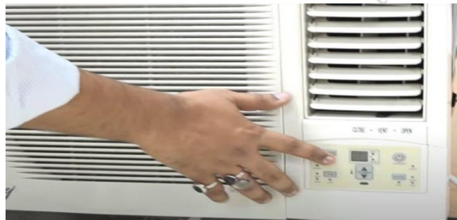
Fig. 1.10 Control panel of window air conditioner
