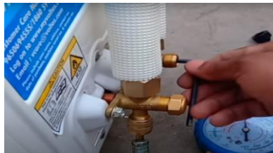
Fig. 2.68 Operating the discharge value using the allen key
