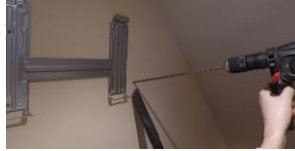
Fig.2.21 Angle downward while drilling
