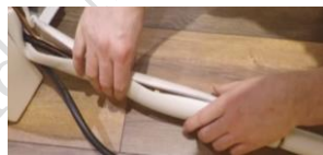
Fig. 2.50 Proper insulation of the both the copper pipes
