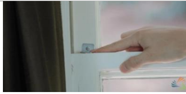
Fig. 2.80 Placement of L bracket
