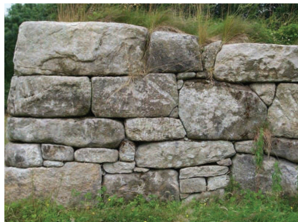
Fig. 1.12: Dry Rubble Masonry
