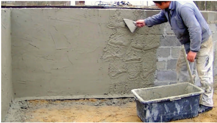
Fig. 3.3: Plastering with manual labour
