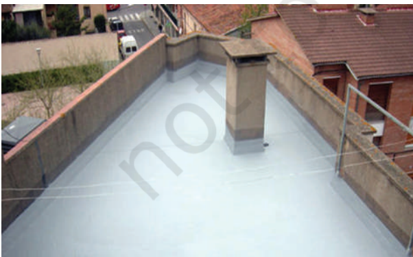
Fig. 5.15: Polyurethane Liquid Membrane
