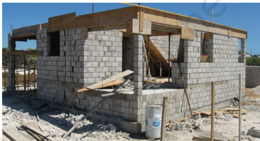
Fig. 4.12: Concrete block wall in house construction
