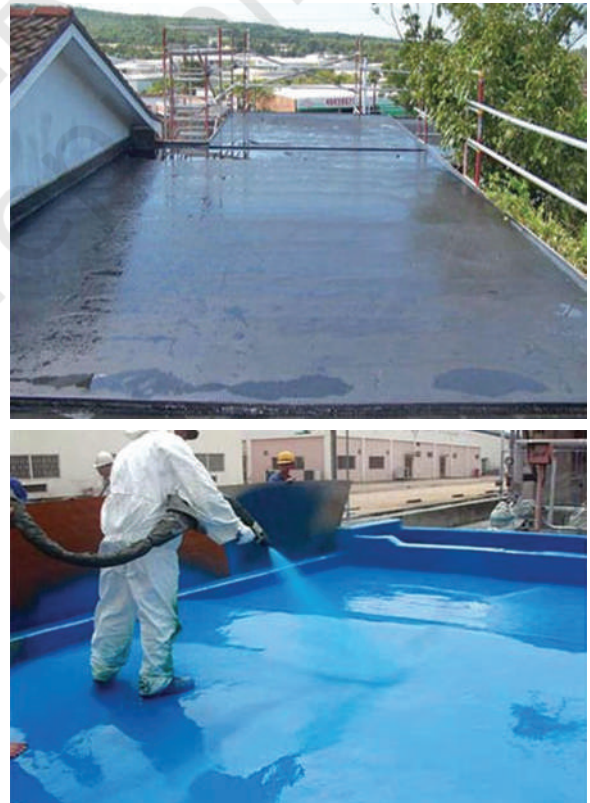
Fig. 5.17: Poly Acrylic chemical coating waterproofing
