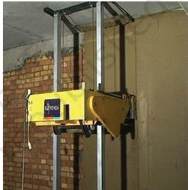
Fig. 3.2: Plastering with machine
