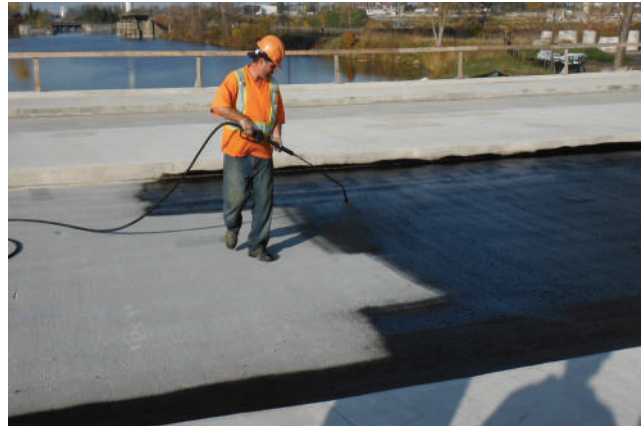
Fig. 5.9: Spraying waterproofing material
