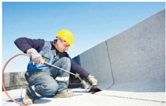
Fig. 5.2: Execution process of waterproofing works
