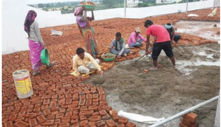
Fig. 5.16: Brick Bat coba waterproofing
