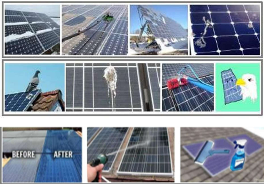
Fig. 12.2: Clean without stepping on the panels or placing heavy objects on them
