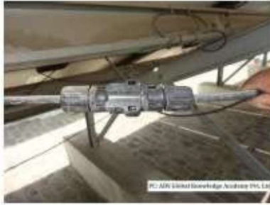
Fig. 8.11: Module interconnection
