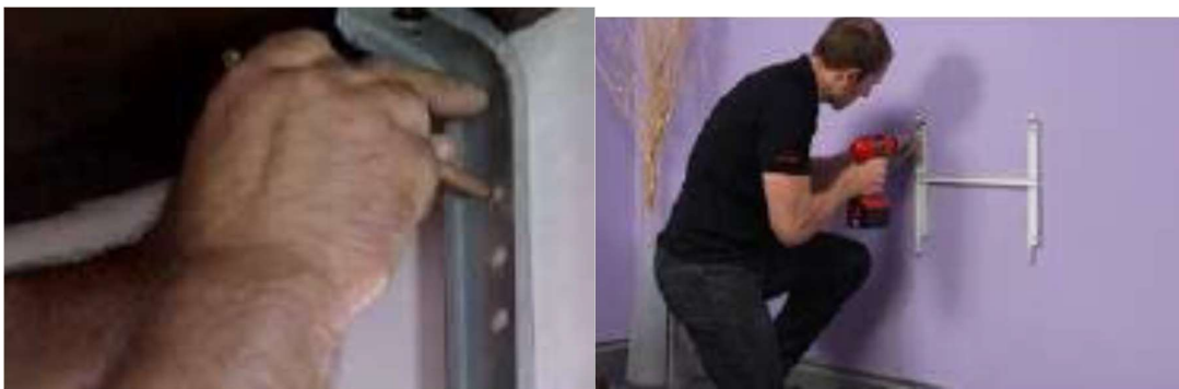
Fig. 8.10: Installation of Inverter mounting structure
