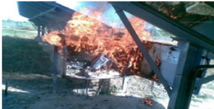
Fig. 9.12: Fire breaking out at the site of a solar PV system
