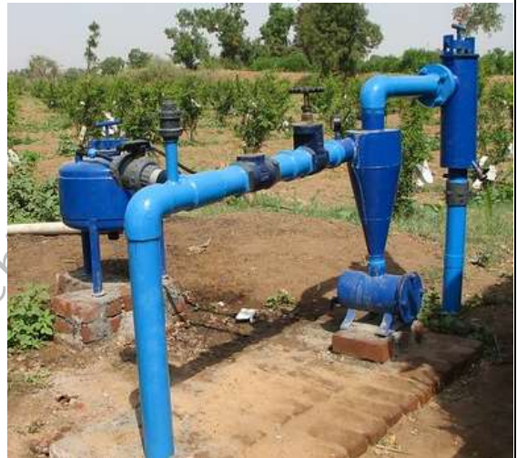
Figure 1.1: Control head
