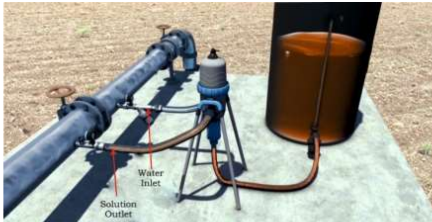
Figure 1.50: Fertiliser injection pump
