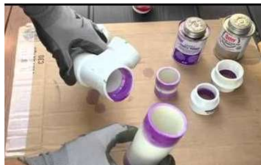
Figure 1.36: Joining pipe and pipe fittings
