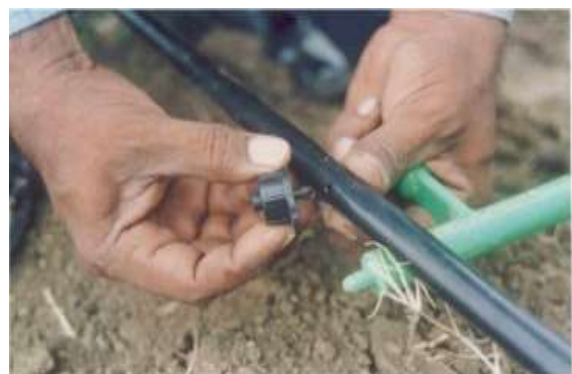
Figure 1.37: Making hole in lateral
