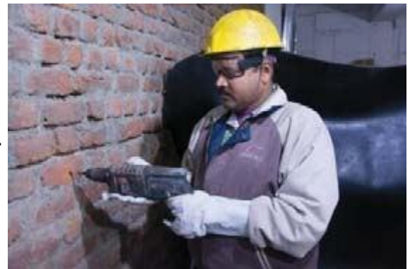
Fig 3.1 Using power drill machine
